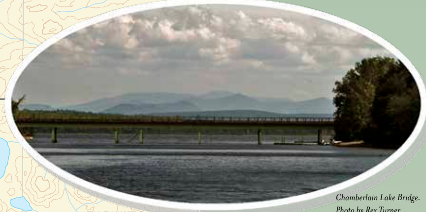
Chamberlain Lake Bridge. Photo by Rex Turner.
